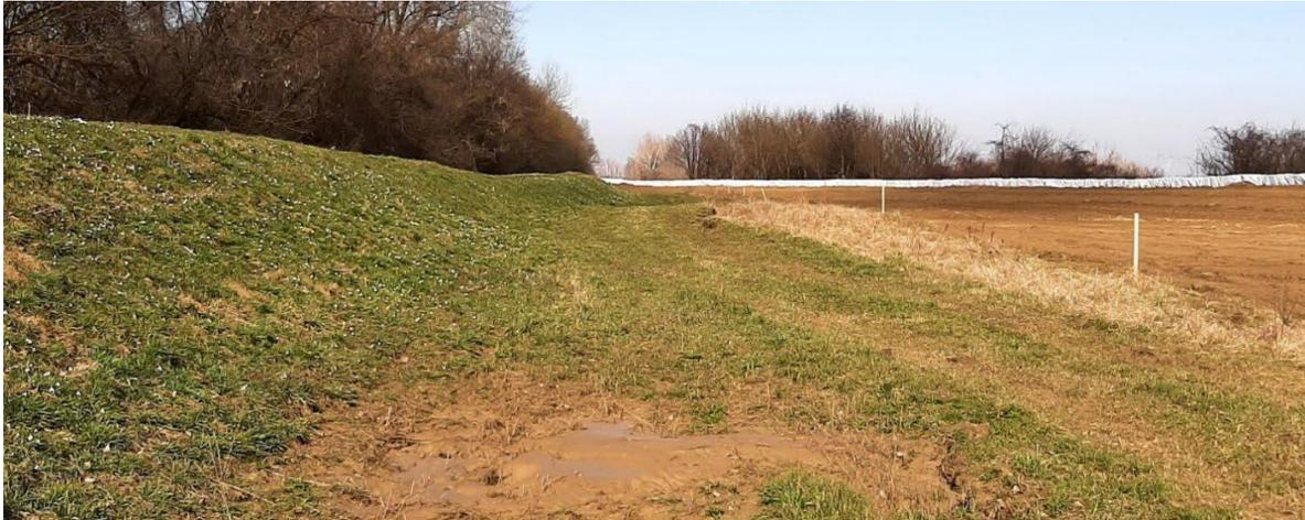
**Figure 1.4** Levee south from Stara Drenčina, along the Kupa river. Sand ejecta are visible in front, levee on the left, settlement of the levee in the distance, and secondary levee (white box barrier) on the right side of the photograph (45.4609N, 16.3362E).
