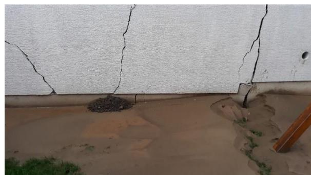
**Figure 1.6** A crack in Brest Pokupski which opened through several yards and houses, ejecting water and sandy soil in time of the main shock (**left** 45.4553N, 16.2628E; **right** 45.4539N, 16.2611E; photos by Igor Gukov).
